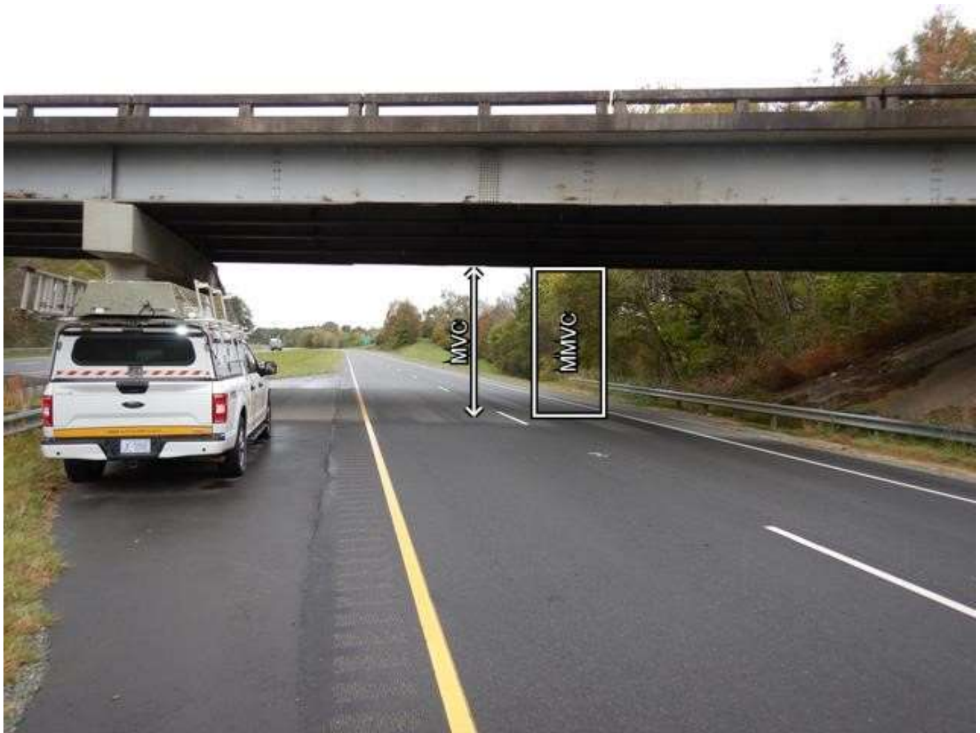
SPAN 2, LOOKING NORTH AT US421NB
