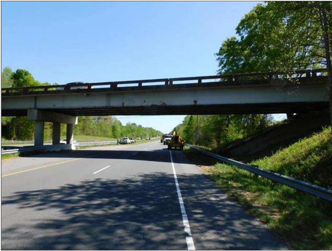
LOOKING SOUTH THRU SPAN 1
