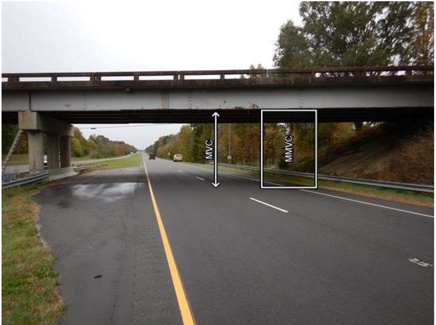
SPAN 1, LOOKING SOUTH AT US421SB
